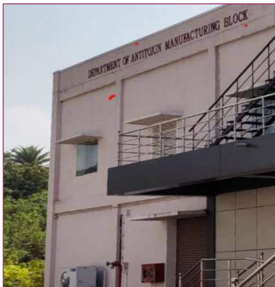
Exhibit 3.1: Newly constructed DAT building
