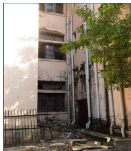
Exhibit 2.24: Leaky sewer lines in Chepauk campus
