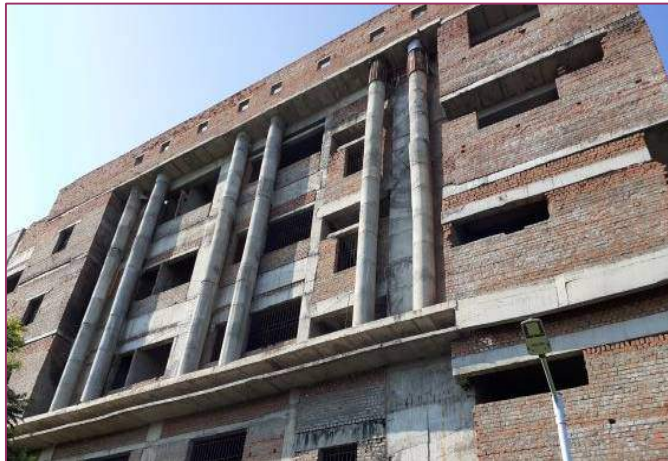
Exhibit 2.20: Facade of the incomplete building
