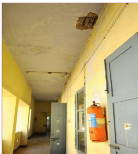
Exhibit 2.23: Damaged roof and time expired fire extinguisher
