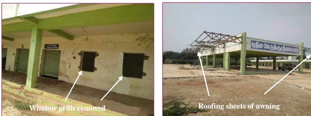
Exhibit 3.7: Damages caused to the asset
