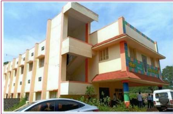
Exhibit 3.9: Full view of the Multipurpose hall
